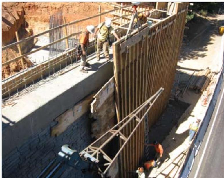
*This photo depicts an incorrect application of a personal fall arrest system—no harness, lanyard, or anchorage point—a violation of OSHA standards.*
